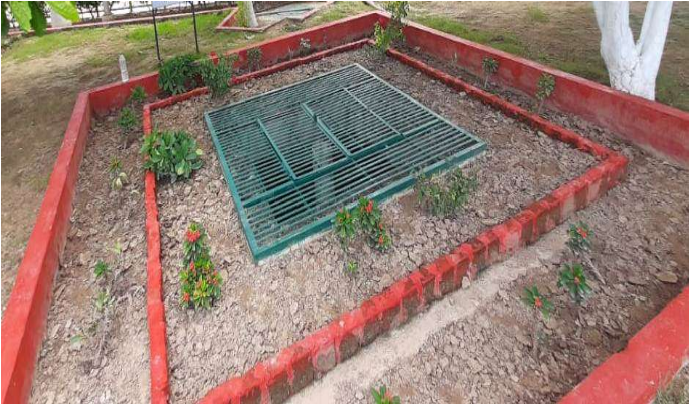
An Example of Rain Water harvesting underground well which may be constructed in GC Dera Bassi Campus
